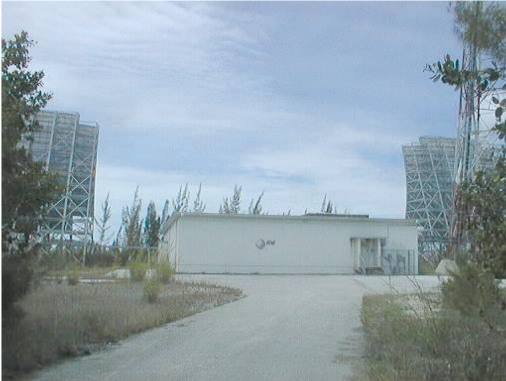
Figure 3. Termination building for offshore cable (TD-2) in Puerto Rico (from Shore.Net, 2009)
