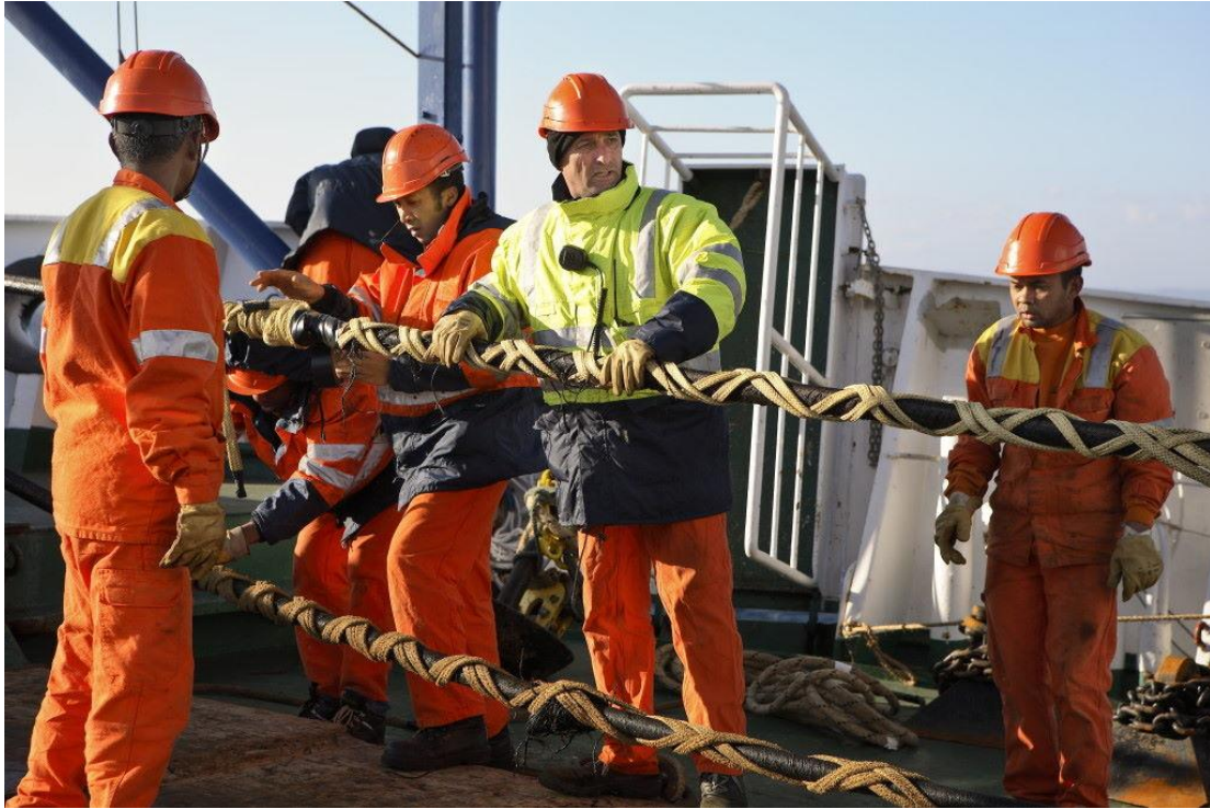
Figure 6. Workers directing cable off ship into ocean (from ISPCPC)
