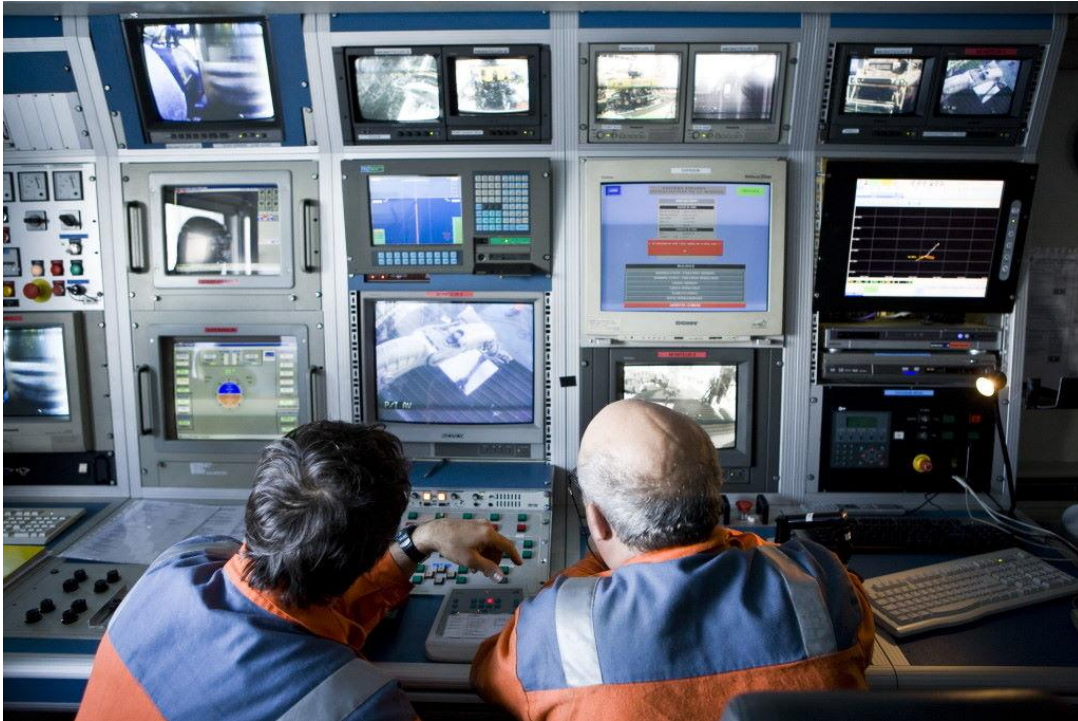
Figure 7. Navigational System in Cable Laying Ship (from France Telecom)
